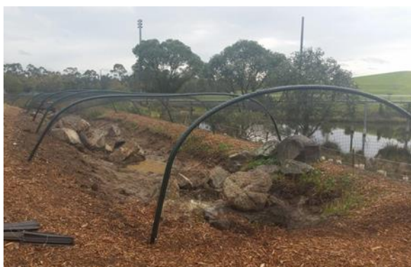
Figure 6 The pond was cleared of excessive plant growth, scraped free of accumulated sediment and netted to prevent bird predation.
