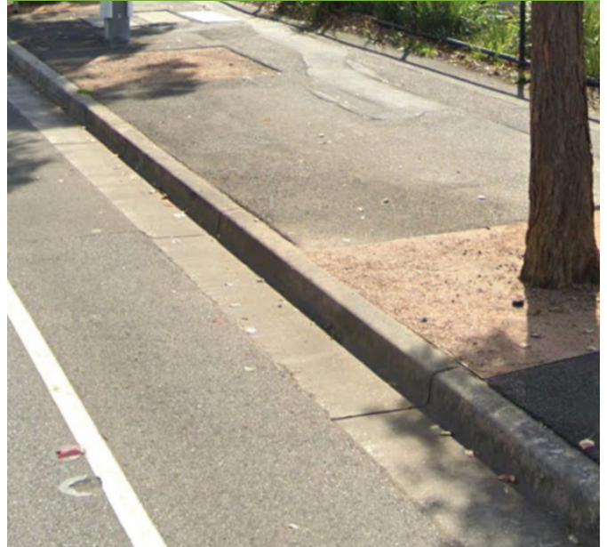
Sample – Insitu kerb & gutter – standard size
