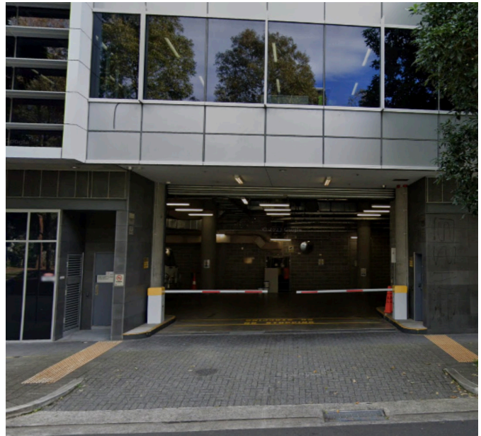
Sample - Brickpave 80 non-interlocking pavement in herringbone pattern
