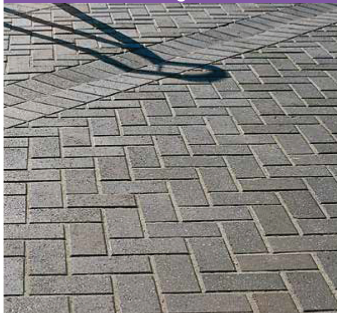
Sample - Brickpave 80 non-interlocking pavement
