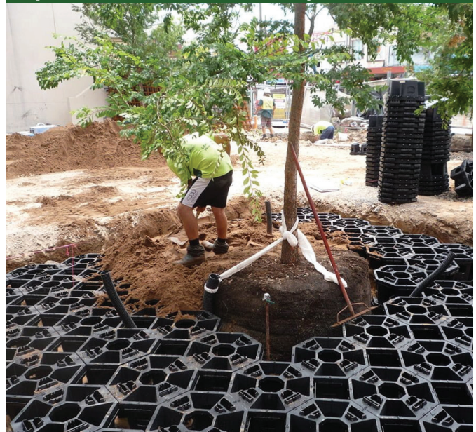
Sample - Tree planting with soil vault system
