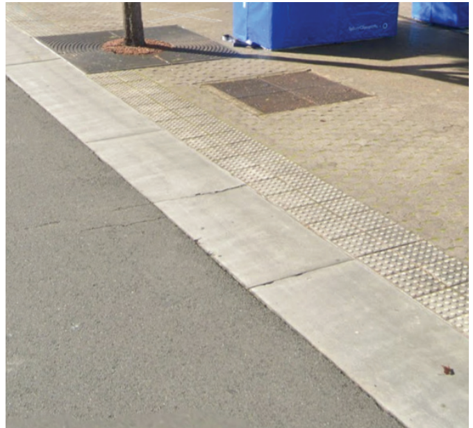
Sample - Insitu flush kerb
