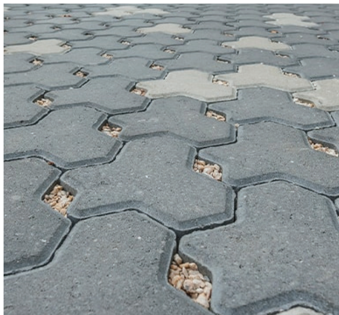
Sample – Ecotrihex 80 permeable pavement
