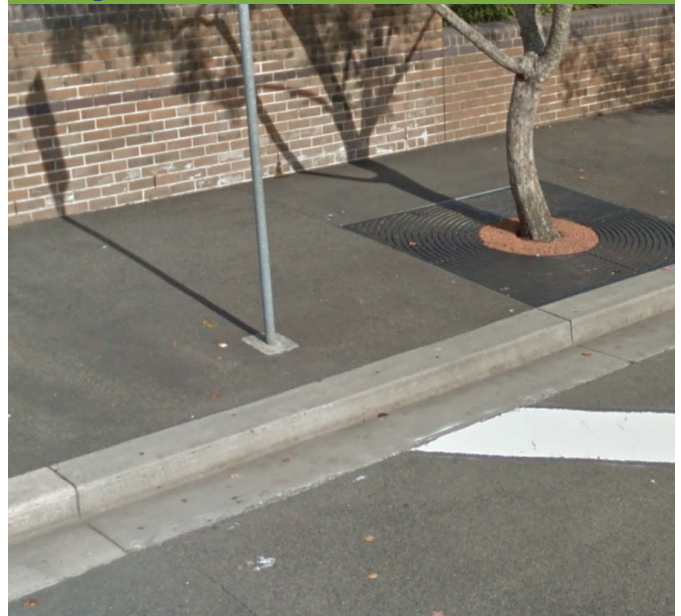
Sample – Insitu kerb & gutter – large size
