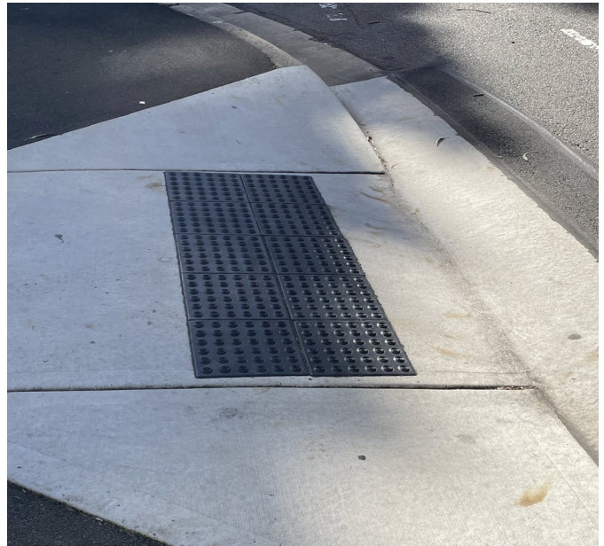
Sample - Standard kerb ramp
