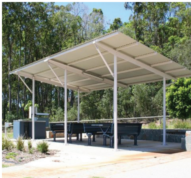
Sample - Picnic shelter
