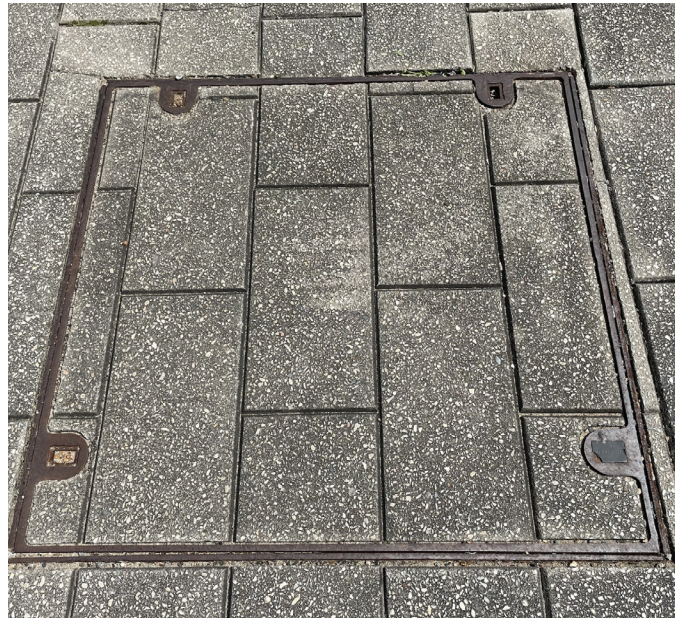
Sample - Single part infill pit lid
