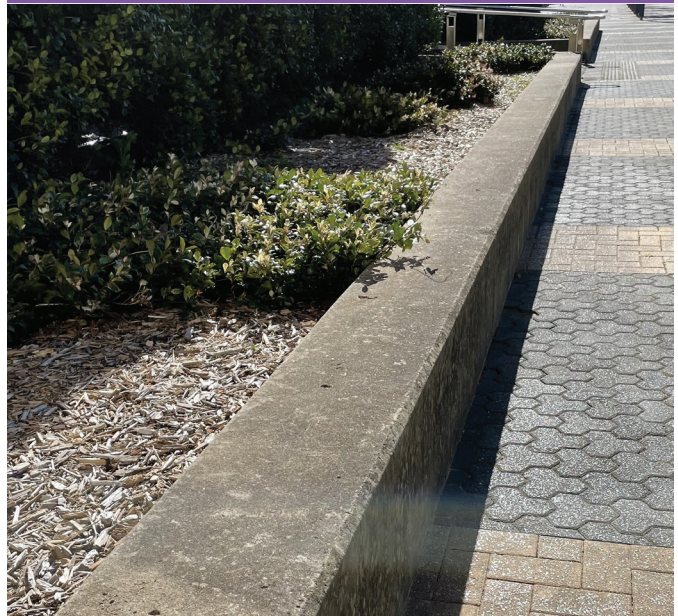
Sample – 400mm Wide Insitu concrete wall
