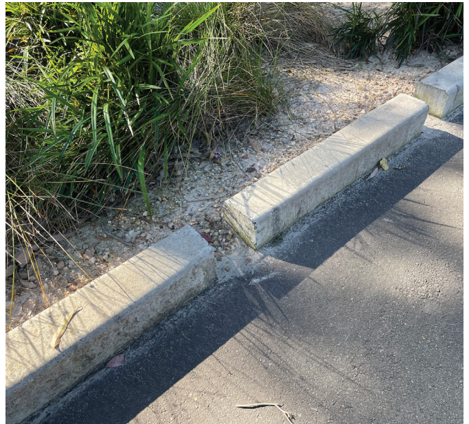
Sample - Permeable kerb
