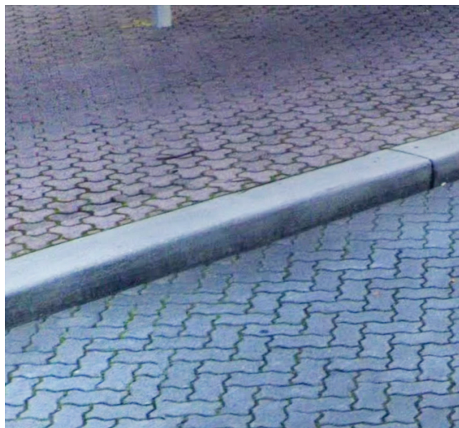
Sample - Precast raised kerb
