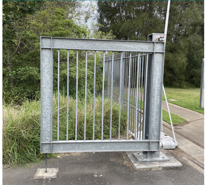
Sample – Palisade fence vehicle gate
