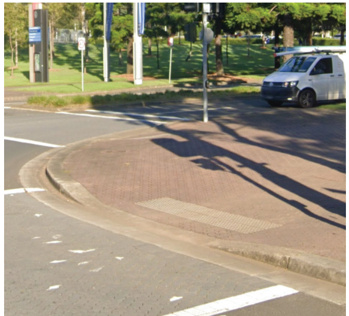
Sample - Large kerb ramp
