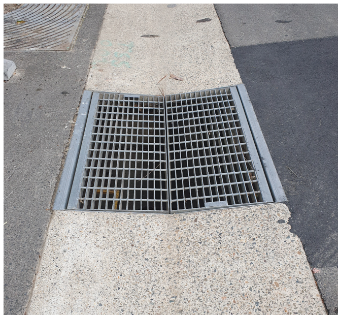
Sample - V-drain swale
