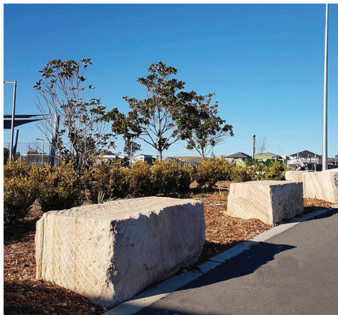
Sample - Sandstone vehicle barrier
